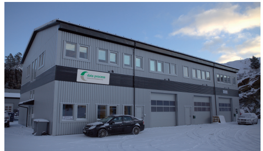
Branch Office Bergen
